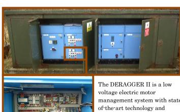
management system with statenetwork communication capabilities that provides Anti-Ragging functionality to wastewater pumps.
